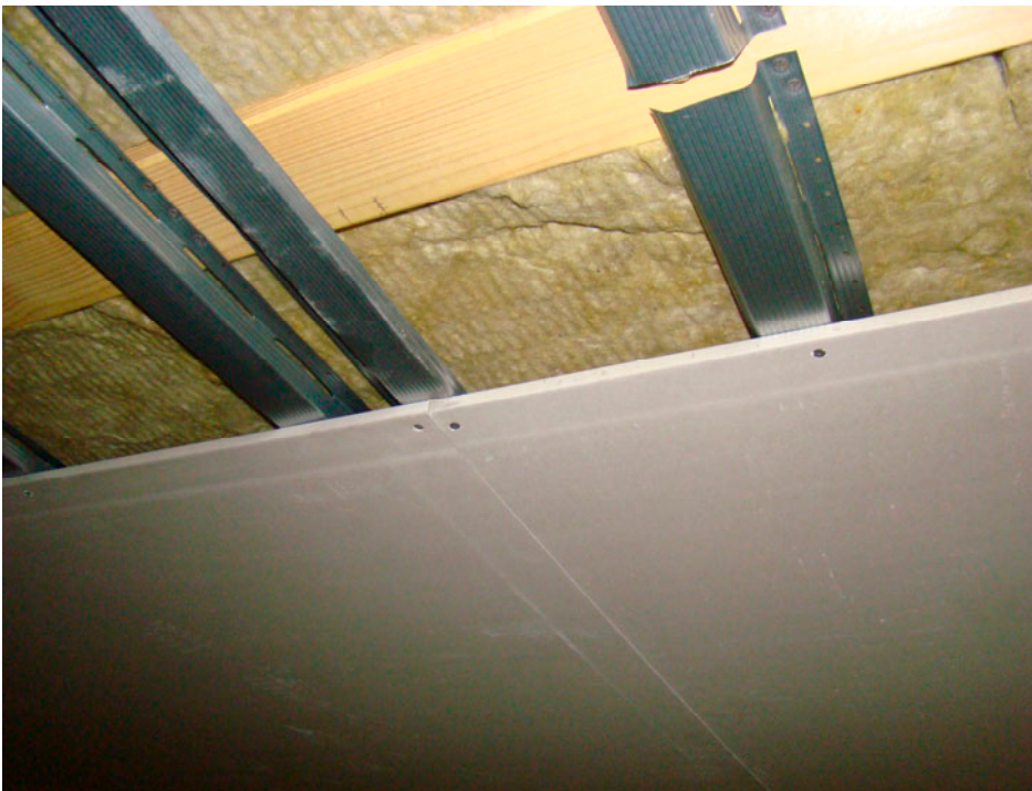
Photo 2 : detail of the mounting of the ceiling channels
