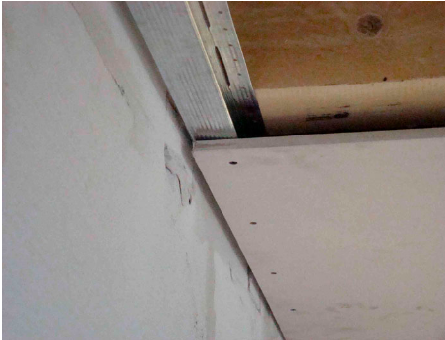
Photo 3 : detail of the mounting of the gypsum boards
