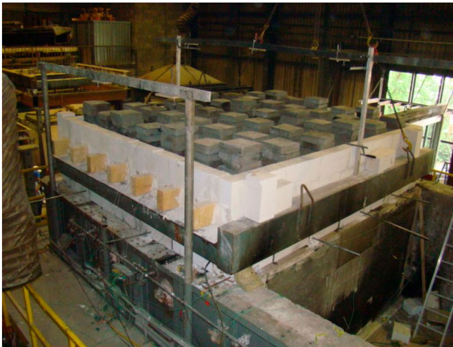
Photo 4 : view of the construction before the test
