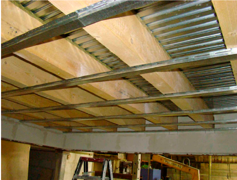
Photo 2 : detail of the mounting of the ceiling channels
